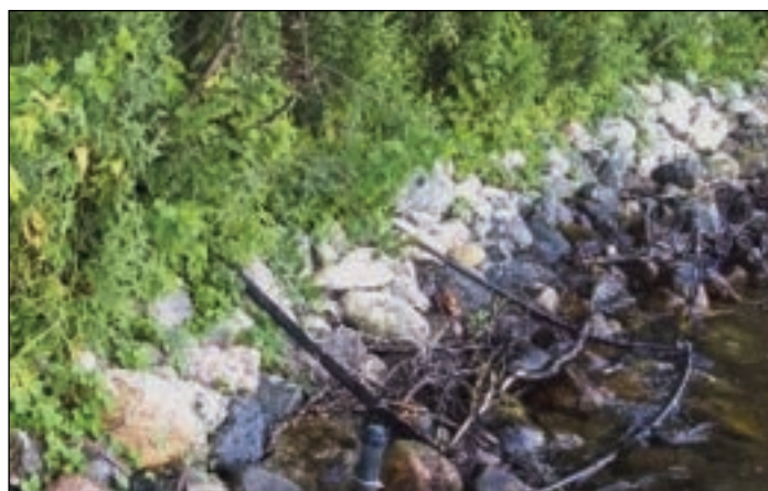
Note the vegetation in and around the rock. Vegetation cannot be removed to place rock. This is the case below and above the OHWL. Vegetation will help hold rock in place, especially in areas that are steep or prone to ice action.
