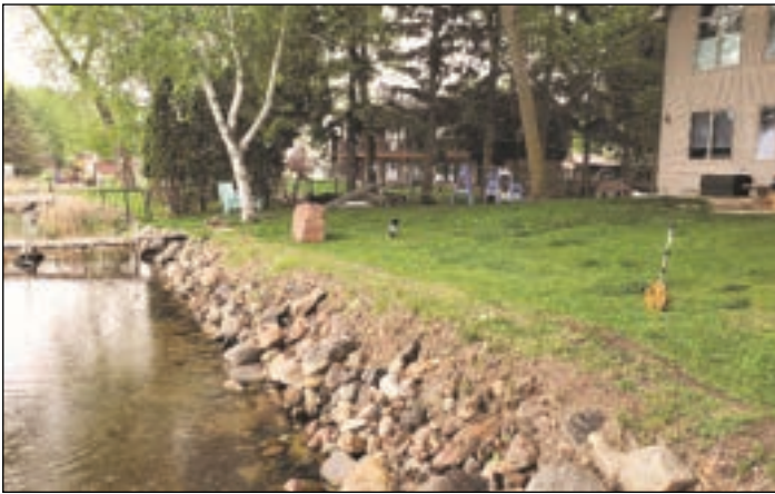
Shoreline with no native vegetation & steep bank. Re-grading & removal of material to make the slope more gradual and establishing native vegetation will improve shoreline stability. Rock can remain at the toe of the bank.
