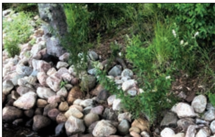
Note the vegetation in and around the rock. Vegetation cannot be removed to place rock. This is the case below and above the OHWL. Vegetation will help hold rock in place, especially in areas that are steep or prone to ice action.
